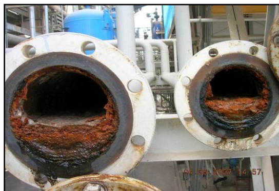
Fig. 6 Fouling effect in the pipe line of gas sweetening plant (ARIANA, 2010; Internet, 2010a, 2009).
